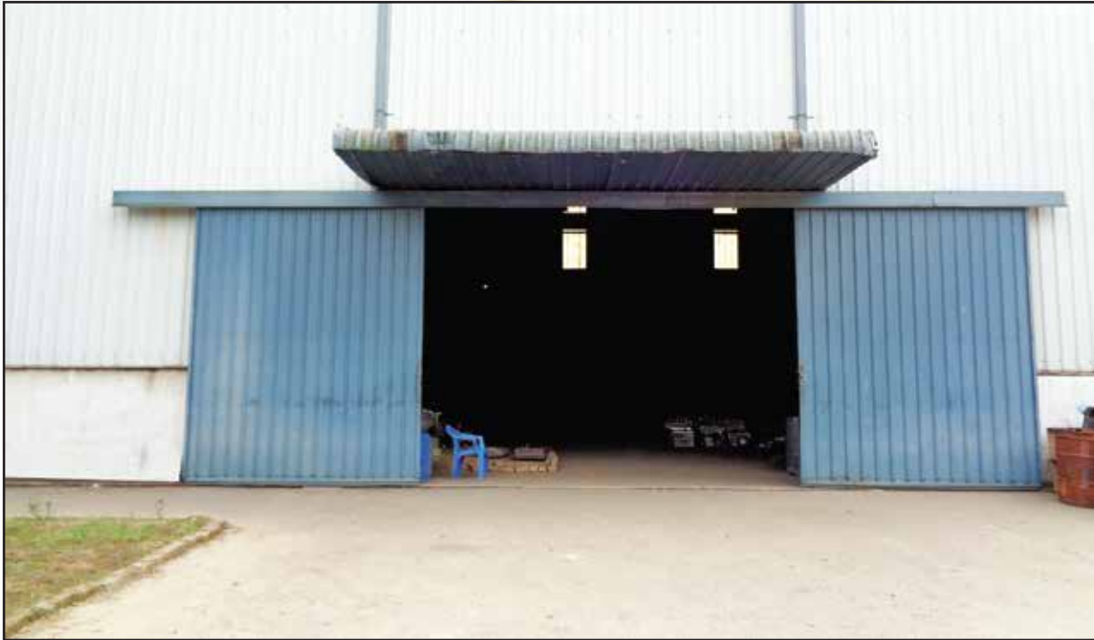
Inside Production House
